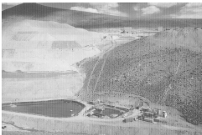
Fig. 1. A large gold leaching operation high in the Andes Mountains at Choquelimpie, Chile. The plastic-lined ponds handle pregnant and barren leach solutions (All figures courtesy Kappes-Cassiday Associates, Reno, USA).
