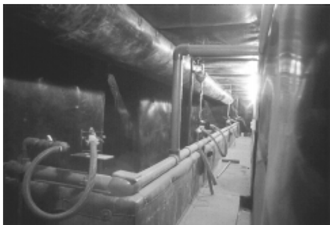
Fig. 5. Interior of Itos plant, Bolivia, showing stainless steel and nonmetallic piping and vessels required to handle hot corrosive leaching solutions. Modern materials make possible handling of fluids that formerly could not be economically contained.
